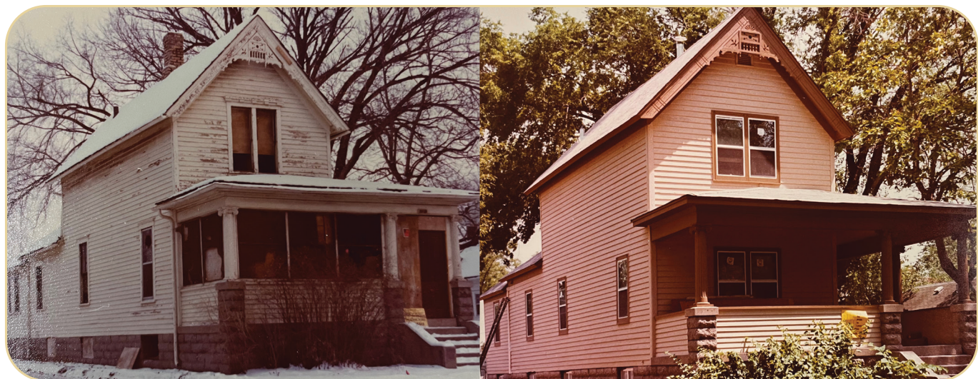
House rehab before and after
